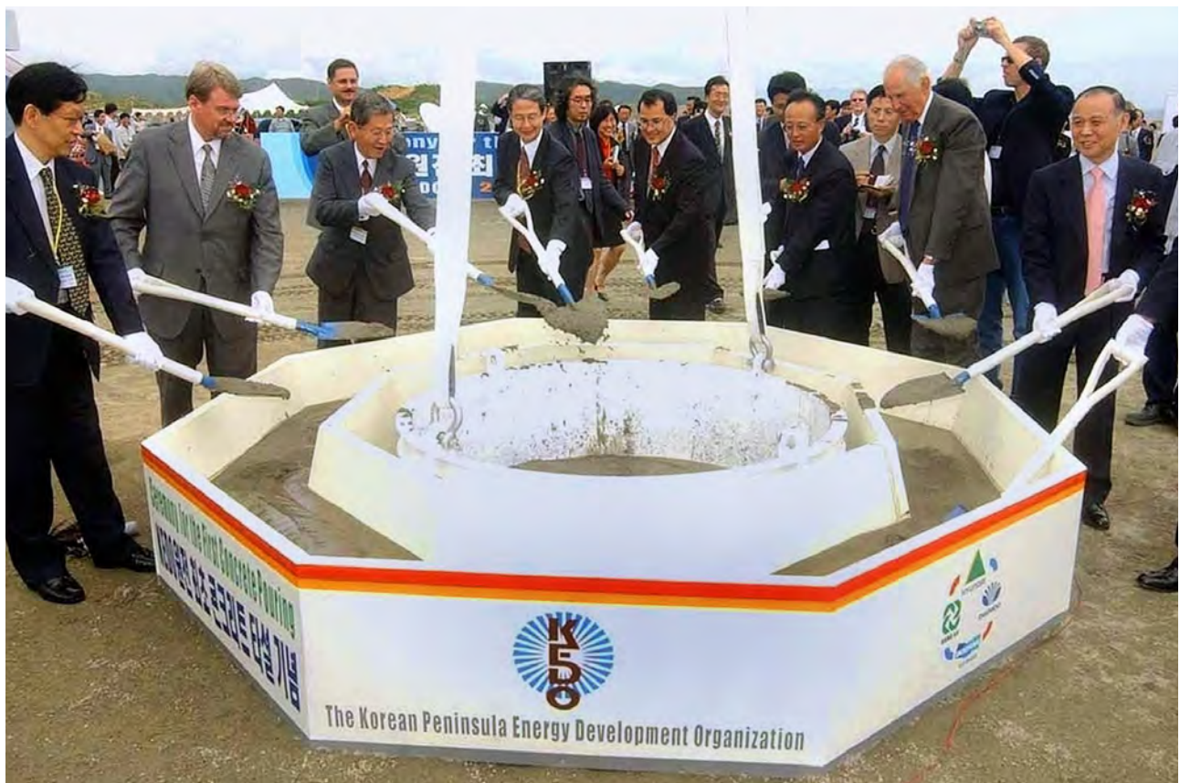
Officials of the Korean Peninsula Energy Development Organization (KEDO) place the first concrete for the foundation of a light water reactor in Kumho, North Korea in August 2002. The provision of light water reactors to North Korea was part of the 1994 Agreed Framework. (Photo by AFP via Getty Images)
