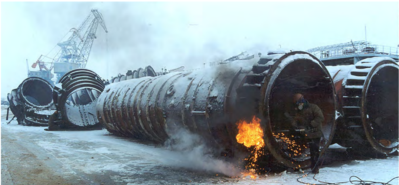
Missile launch tubes removed from a Soviet ballistic missile submarine are eliminated as part of the Department of Defense's Cooperative Threat Reduction program in January 2010. This program could serve as a model for dismantling North Korea's nuclear weapons program. (Photo by Defense Threat Reduction Agency)
